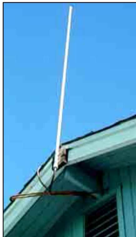
Figure 5—The completed antenna mounted to the roof.
